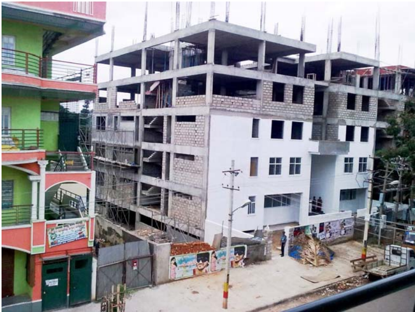
View of the building from Sirsi Road
